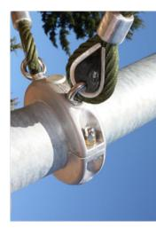
Corocord aluminium clamps are used as connectors between steel posts and rope. Two aluminium castings are bolted together. The height of the clamps is thus variable.
